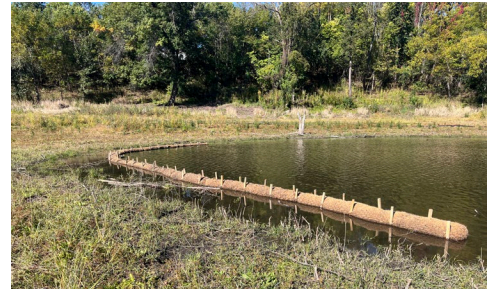
Coir logs installed along the shoreline of Seidls Lake
